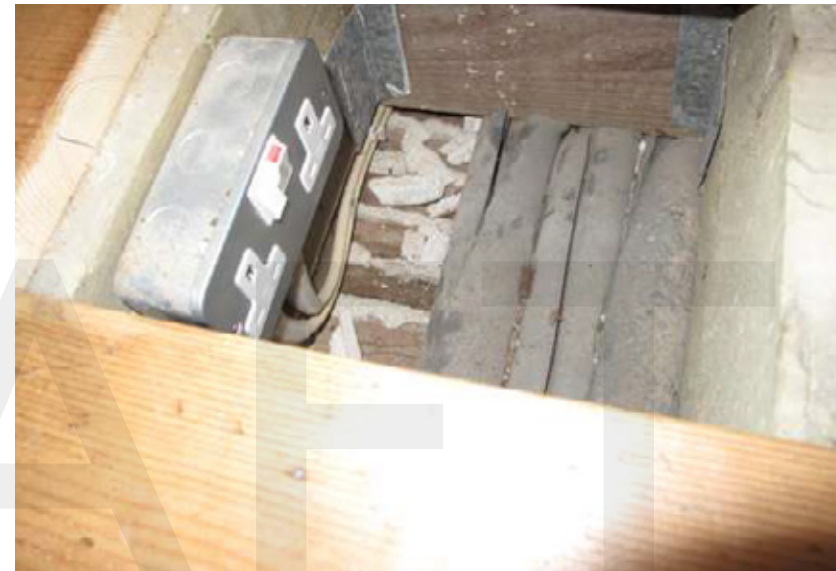
10. View into access point showing plaster debris from damaged key to timber
