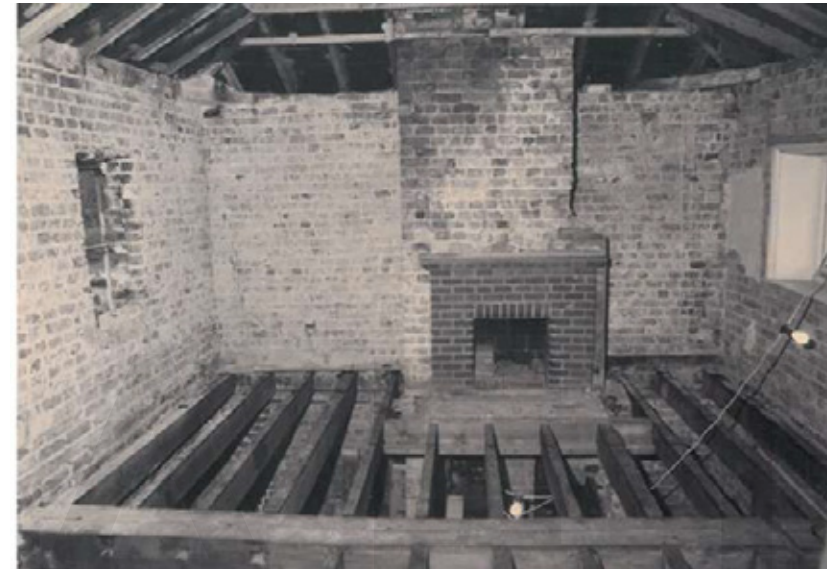
Record photo from 1990. First floor north wall
