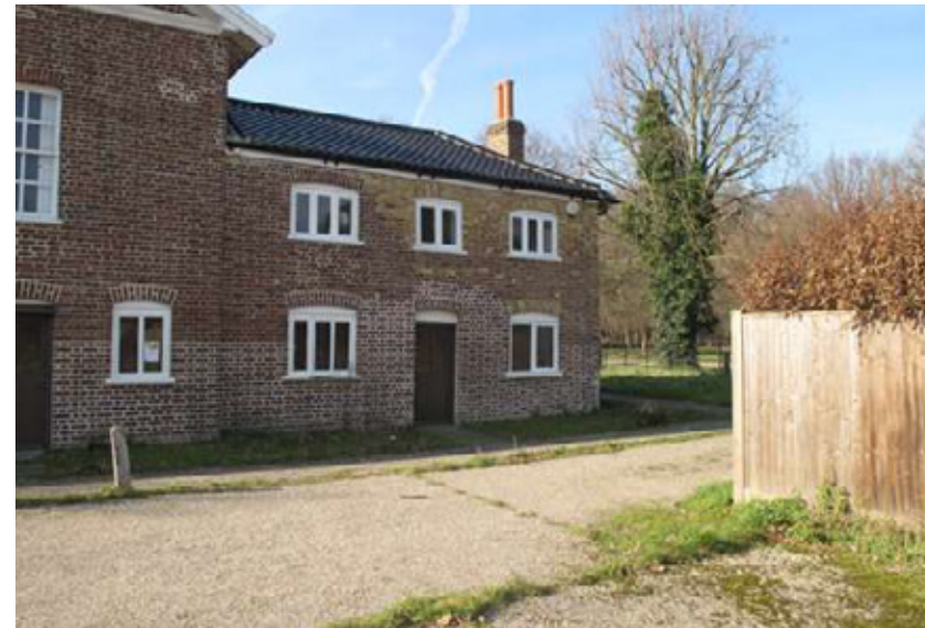
4. East elevation showing areas of previous work to the brickwork
